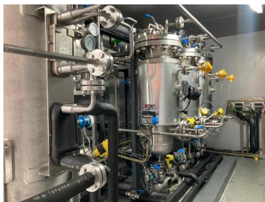
Figure 3. H 2 deoxidation and drying system
